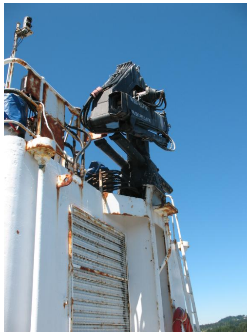
Figure 8: Stores crane and aft bhd of emerg. gen. compt. on boat deck
