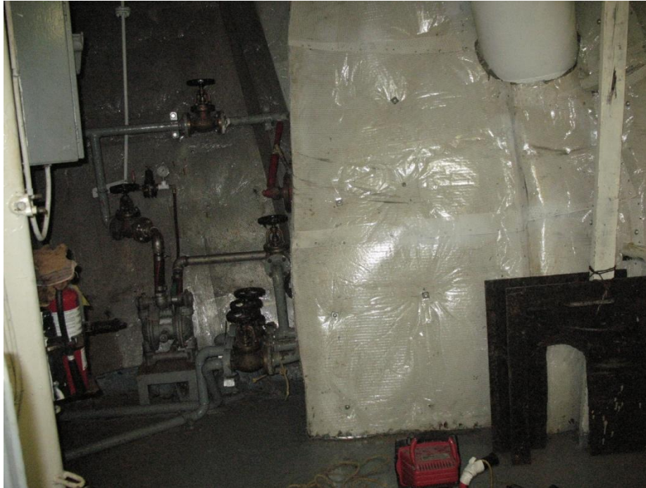
Figure 15: Foc'sle interior, looking at the port anchor pocket
