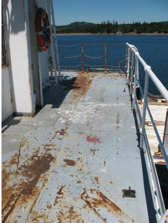
Figure 5: Upper deck, port side looking aft
